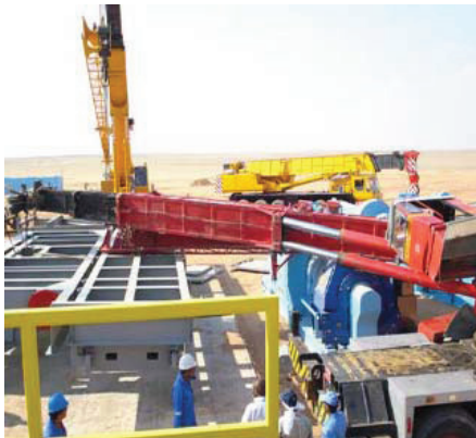
Upper crane structure (operator cabin, crane boom telescopic sections) fell across the drawworks platform and struck the drawworks brake cover.
