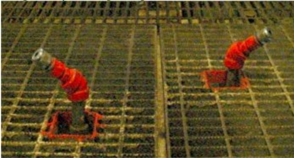
Deluge head protruding through deck
