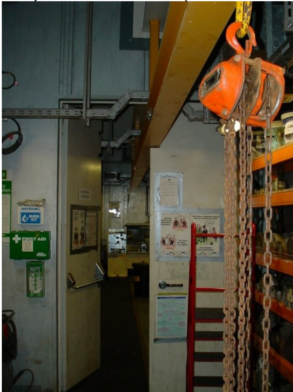
Runway beam from mechanical workshop into fabrication workshop
