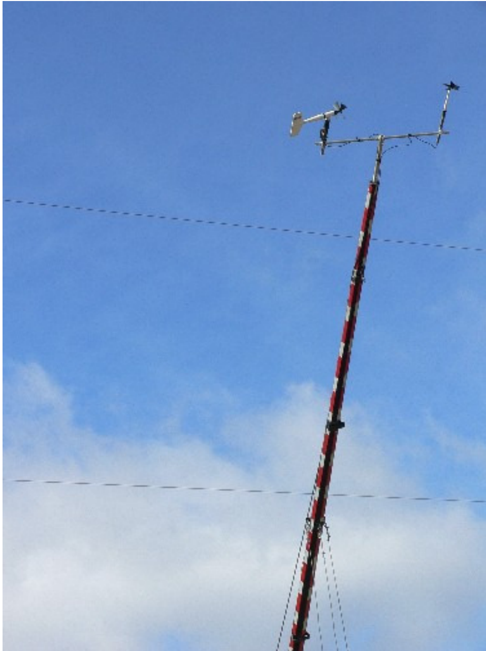
MET Tower in Contact with Power Lines
