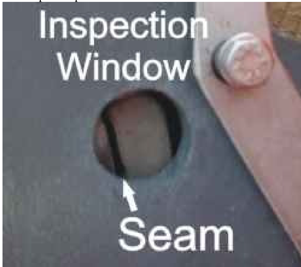
Close-up of Inspection Window and Seam
