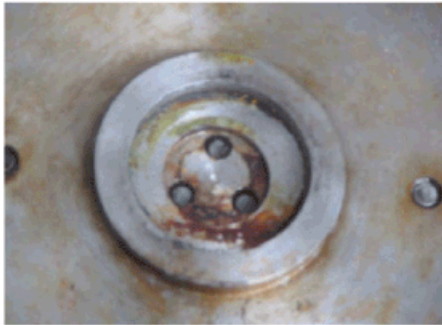
Pict 12. 30 kg camera is supported 3 off 6 mm bolts.
