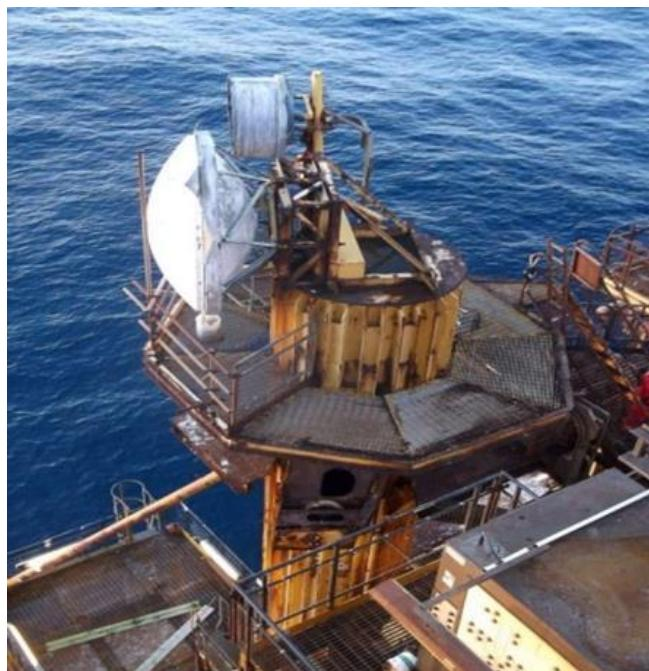
View of crane pedestal from above showing the perimeter walkway after guardrails had been removed
