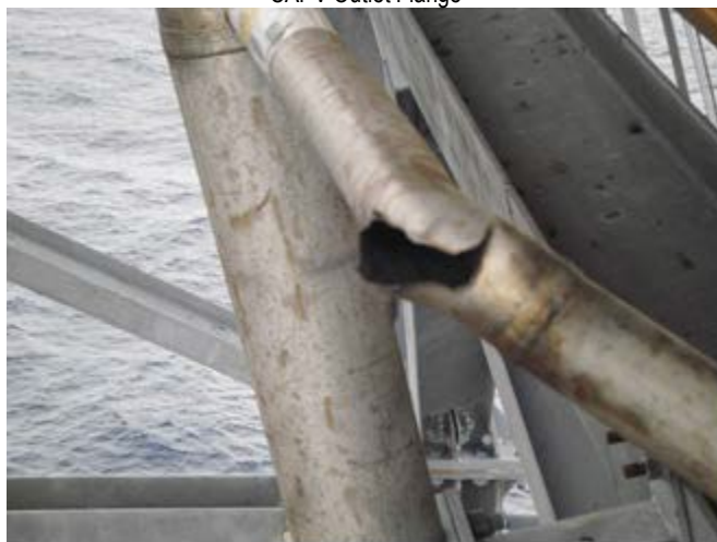
Ruptured Interconnected Pipe
