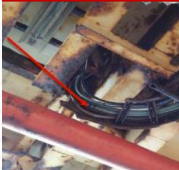
Potential dropped Object: – Piece of ladder rack weighing 3kg
